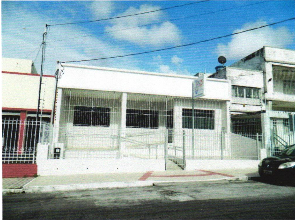
Fachada Principal I
