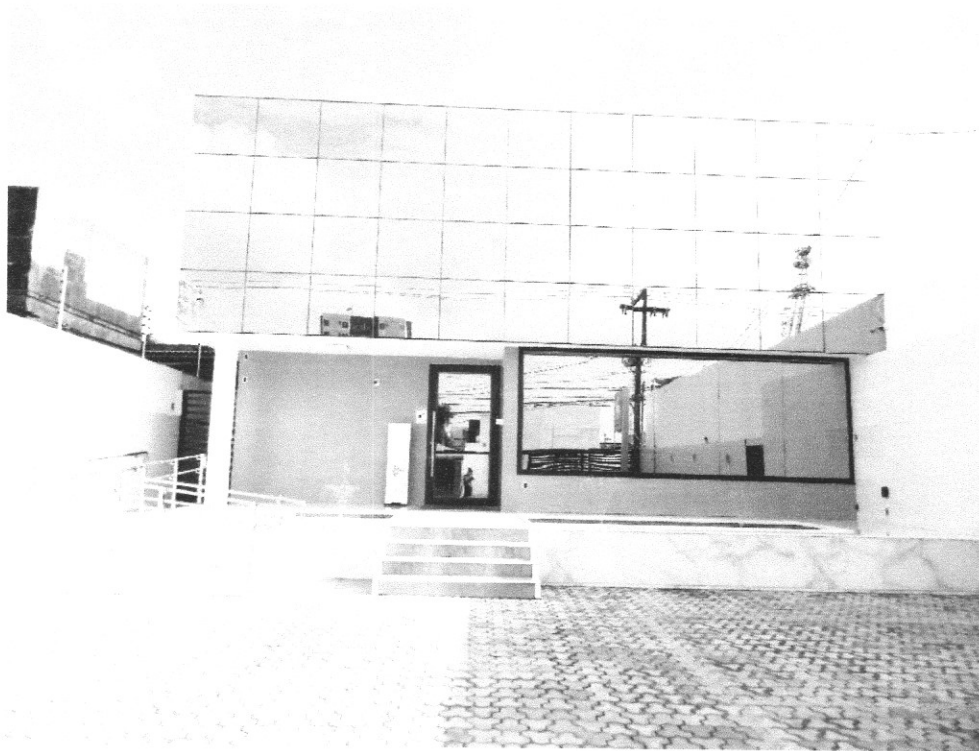
Fachada Principal I
